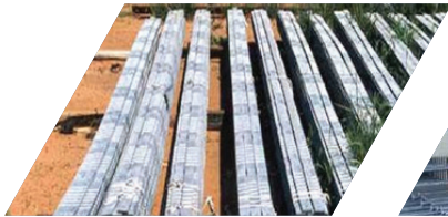
Steel strips reinforcement
