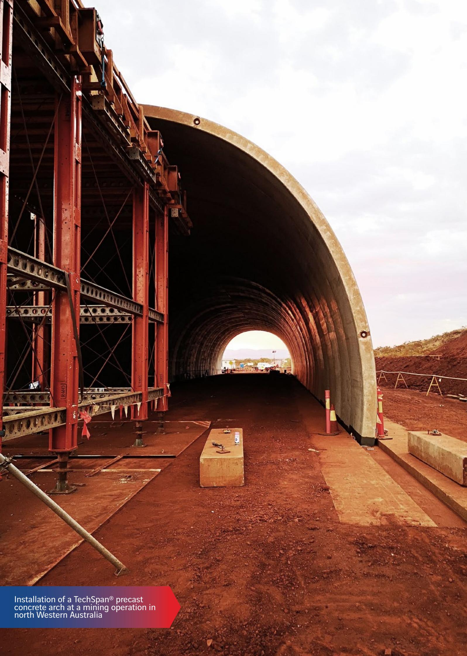
Installation of a TechSpan® precast concrete arch at a mining operation in north Western Australia
