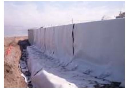
Left: Tierra Armada engineers designed the Reinforced Earth® wall to be raised to almost 22m high in Stage 2.
