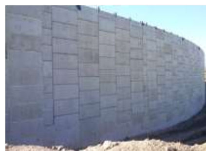
Main Picture: Construction of Stage 1 Reinforced Earth® Walls
